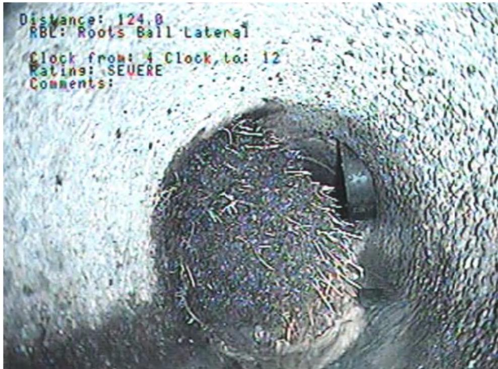
**Example #2 - Pictures of Heavy Debris, Roots and Grease Causing Partial Blockages:**
