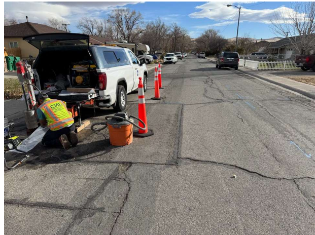
Photograph 6: Pavement Condition at C-24-11
