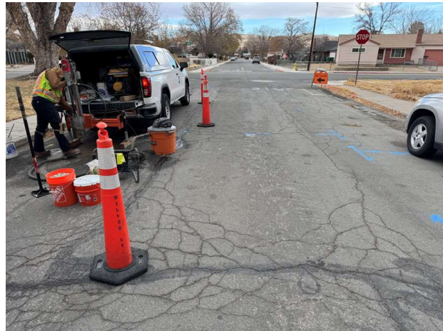
Photograph 8: Pavement Condition at C-24-13
