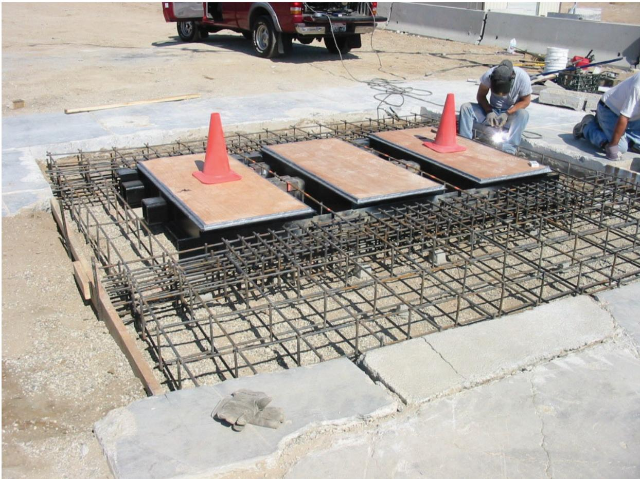
Photo 6 - Three DSC2000 Phalanx Barriers installed on U.S. Department of State spacing of 42 inches [107 cm]. The two rebar beams have been installed and the lighter outer rebar placed about them. All bars are size 4 (0.5 inch [13 mm]). Note that the Barriers are placed directly in the 11 inch [28 cm] deep excavation. Plywood has been placed on the ramp plates to protect the finish from the concrete pour.
