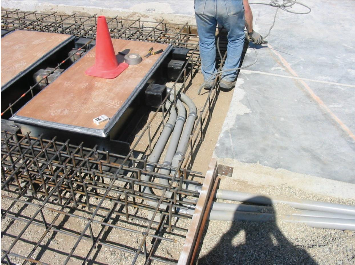
Photo 7 - Three PVC conduits have been installed for the hydraulic hose interconnect. Two of these will run straight through the first Barrier on the way to the second and third Barriers. These ducts should be run in the most direct route possible to the hydraulic power unit.
