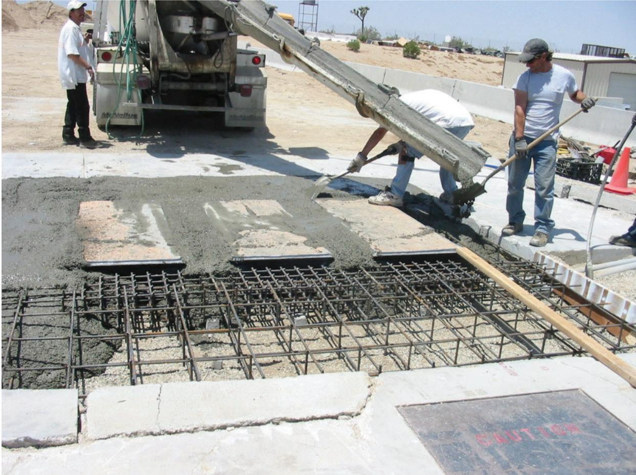
Photo 8 - 3000 psi [20.68 Mpa] transit mixed concrete is being distributed during the pour. All hydraulic hose ducts and electrical conduits have been installed by this point in the installation.
