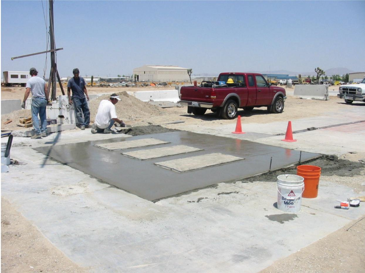
Photo 9 - The concrete has been screeded and tamped. Additional concrete has been poured to patch the other excavations necessary for a complete installation.
