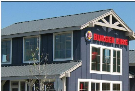
3.3.3.3 a) Exposed rafter ends, overhanging eaves, multiple roof planes and varied fenestration create interesting commercial buildings.
