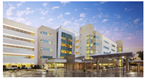
3.3.4.1 a, b) Visual interest and articulated building facades.
