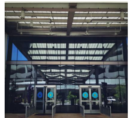
3.3.4.2 a, b, d) Highly visible building entryways with material accents.
