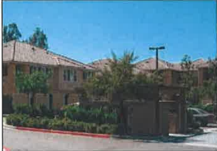
3.2.3.7 a) Trash enclosures with landscape screens and architecture that is similar to that of the project help to minimize the negative visual impact of these structures.
