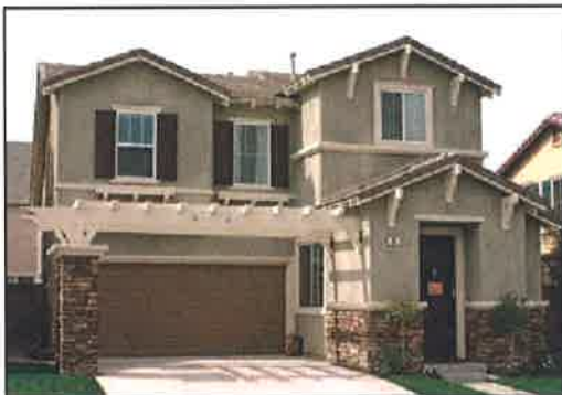
3.3.4.11 a) Recessed garages give importance to the entry and create a pedestrian friendly neighborhood.
