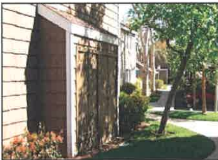
3.2.3.7 d) The screening of utilities can be integrated into the adjacent building through the use of similar materials and architectural elements.
