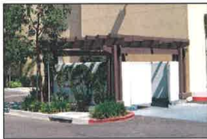
3.2.1.8 d) Screening of refuse containers and utilities is an inexpensive way to maintain the attractiveness of shared open space.
