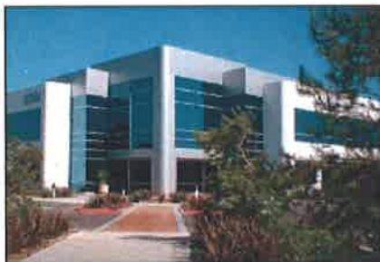
3.3.3.4 b) Quality building materials enhance the look of office/business parks.
