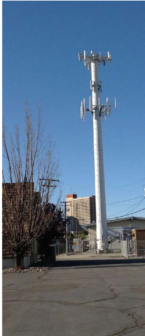
Example of Macro Cell Tower – 106 ft tall
