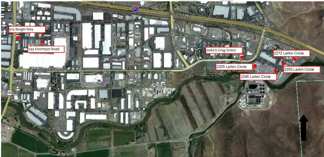
Figure 1: Aerial view of the seven (7) noncompliant structures identified during the CAV.
