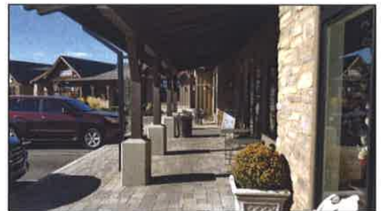
2.5.16 (a)(c) Roof variations and covered entries provide interest and protection from the elements for customers.
