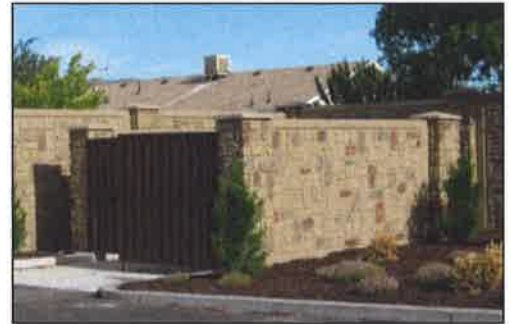
2.3.9 (b) Trash enclosures with landscape screens and architecture that is similar to that of the project help to minimize the negative visual impact of these structures.
