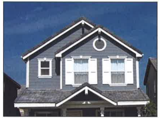
2.4.12 (a) Varied roof planes including shed roof design and second story facade details add visual interest.
