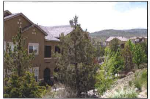
2.3.1 (a) Building setbacks and orientation with landscaping creates visual interest from roadways.
