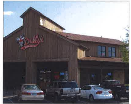
2.5.18 (b) Natural looking materials such as wood add authenticity to buildings
