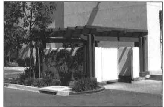
2.5.11 (b) Screening of refuse containers and utilities is an inexpensive way to maintain the attractiveness of shared open space.
