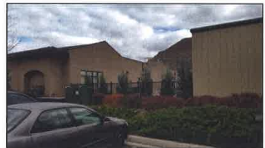
2.5.17 (e) Varied roof designs add to the interest of projects such as this mini-warehouse development.
