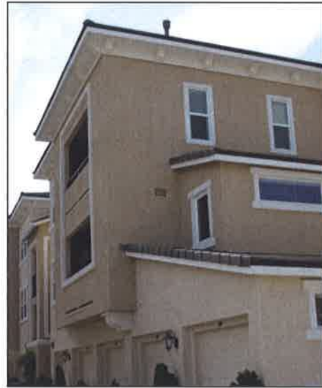
2.3.13 (a)(d) Roof profiles and attention to detail on the underside of eaves enhances cohesive architecture.
