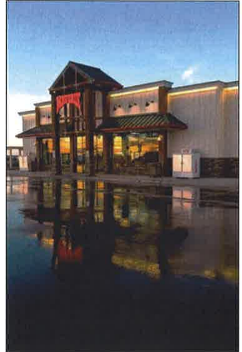
2.5.8 (i)(j)(k) Architectural lighting example provides attractive but not overbearing night lighting.
