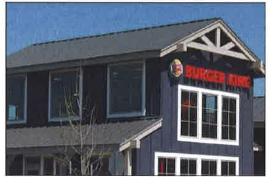
2.5.17 (a) Exposed rafter ends, overhanging eaves, multiple roof planes and varied fenestration create interesting commercial buildings.
