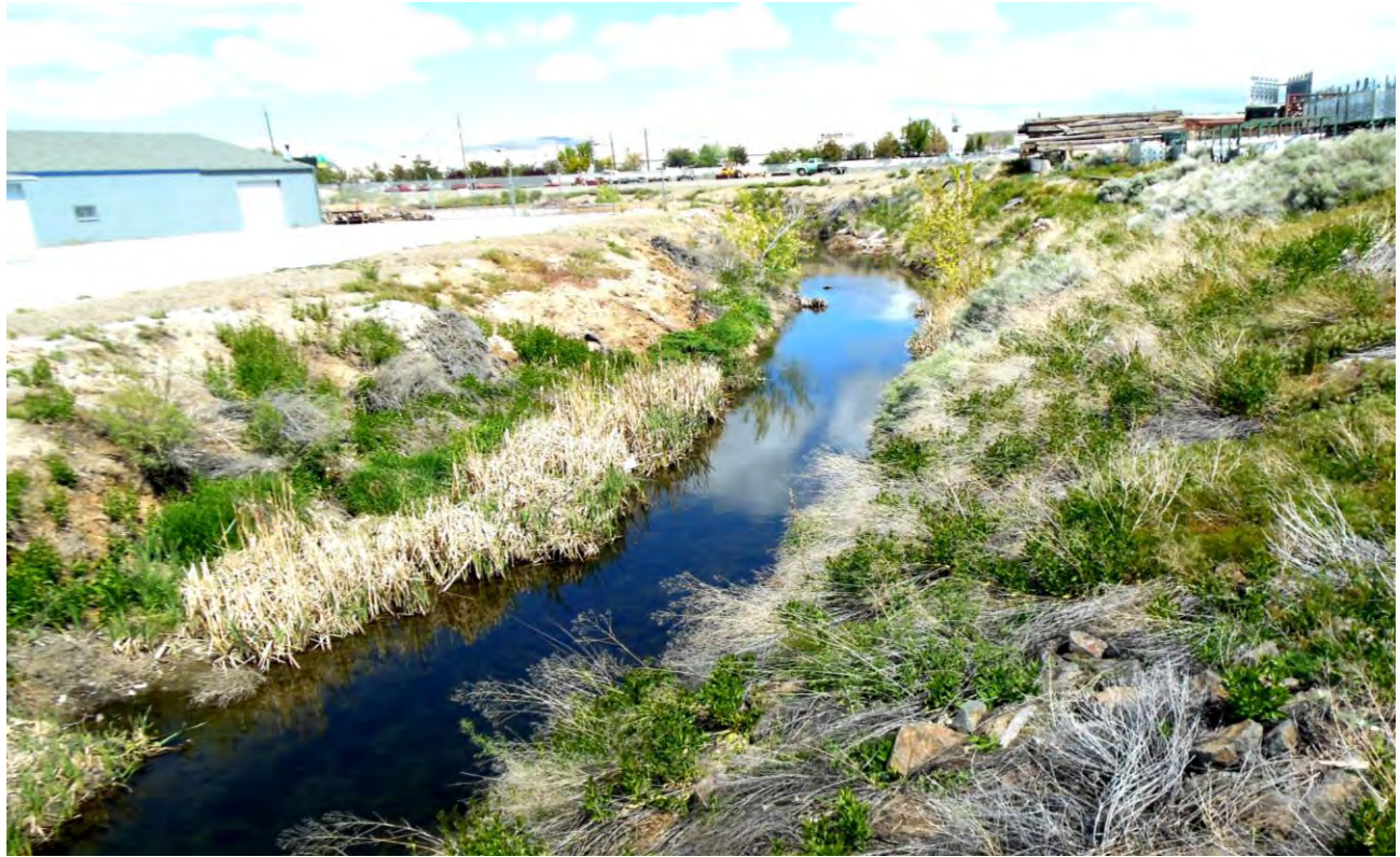
Photo #3: Existing NTD looking north from the Kleppe Lane Bridge
