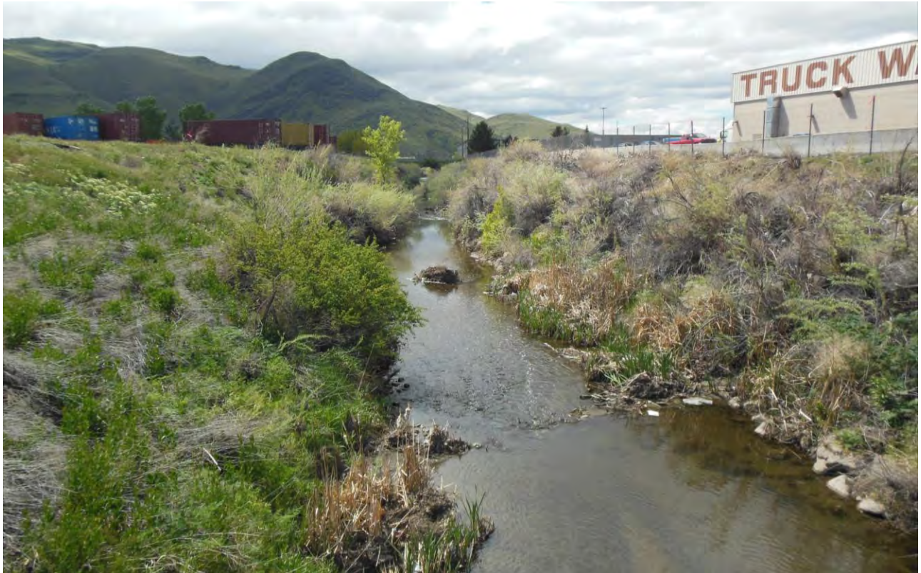
Photo #2: Existing NTD looking south from the Kleppe Lane Bridge
