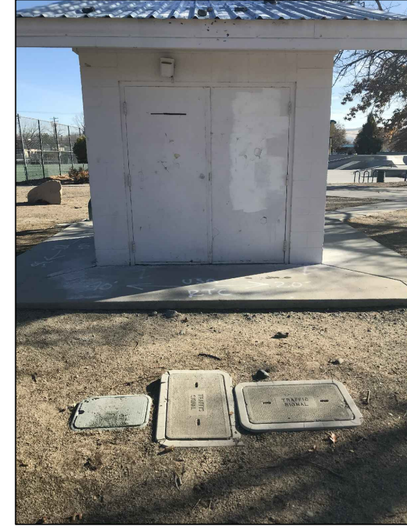
EXISTING N-9 AT RESTROOM
