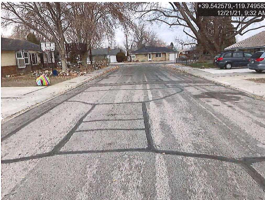
Photograph 1: Typical Pavement Condition for 5th Street from G Street to H Street
